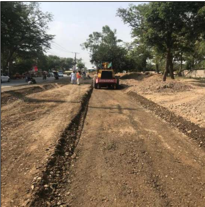
Picture 63: Compaction of widening portion in progress
