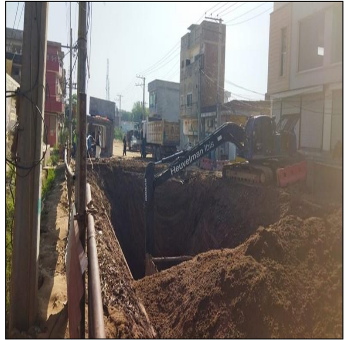
Picture 39: SCC Excavation in Progress @ Marala Road
