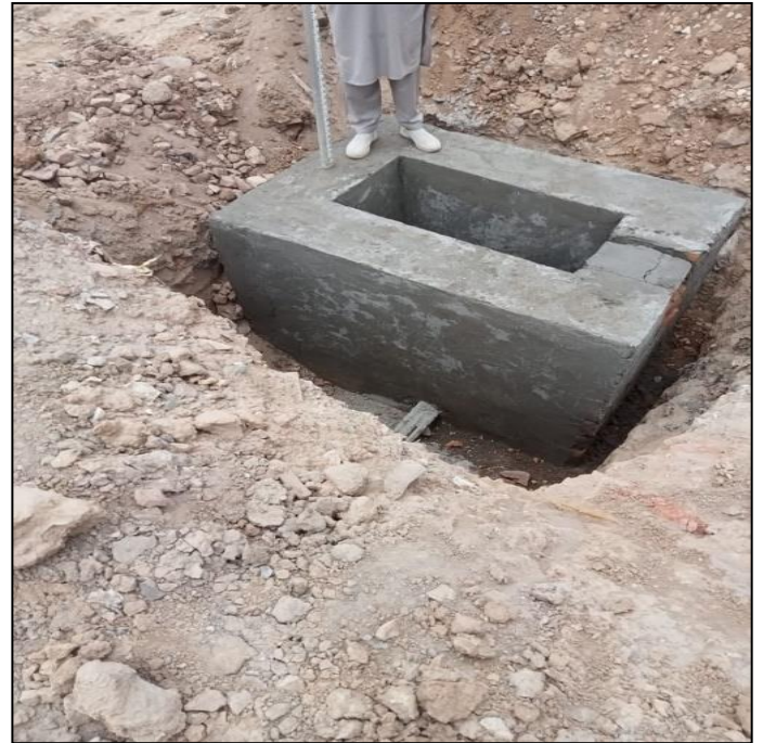
Picture 41: Gating Chamber Work @ Marala Road
