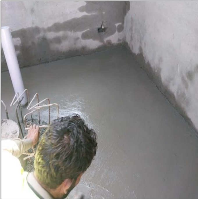
Picture 52: Floor work of New Tube well Pump Room
