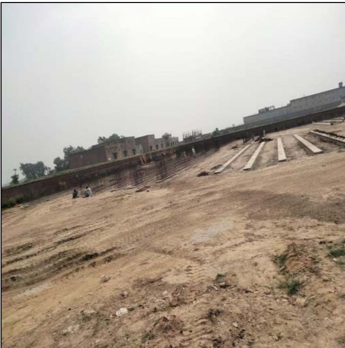
Picture 67: Girder Yard
