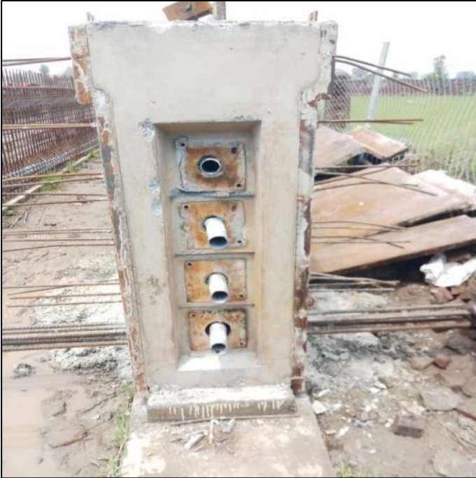
Picture 65: Casting of 2nd girder
