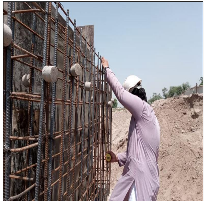
Picture 20: Steel Inspection of Manhole # 64 at Arra Tullah Road.
