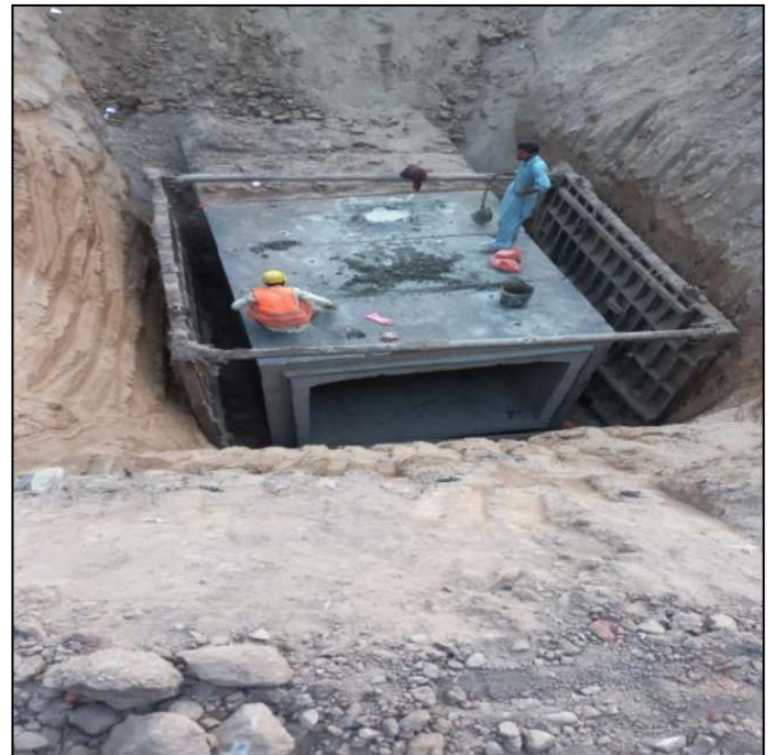
Picture 43: SCC Grouting in Progress @ Marala Road
