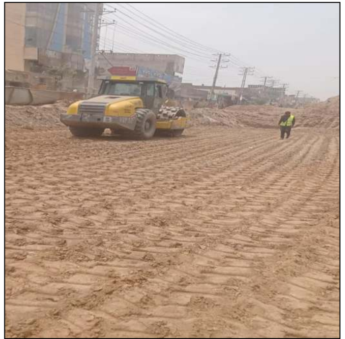
Picture 47: Subgrade Compaction in progress @ Airport Road
