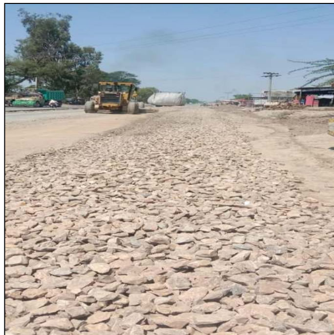
Picture 26: Lot-4 Restoration of Pakpattan Road in progress
