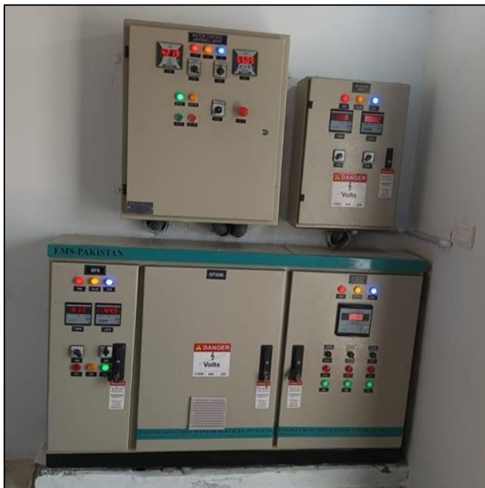
Picture 11: Installation of MCUs and DBs at Pump House Madina Masjid
