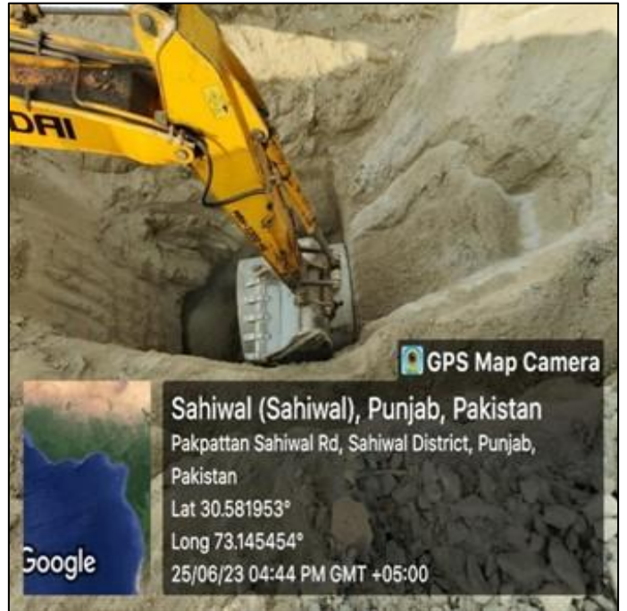
Picture 16: Pipe laying in progress at L-3 Dia 72" Lot-04
