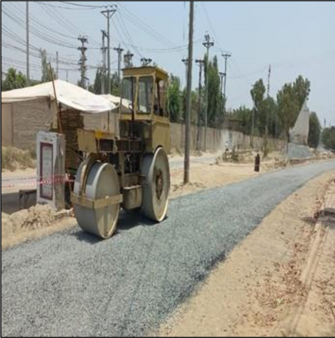
Picture 13: L-2.2 42" dia TST work in progress
