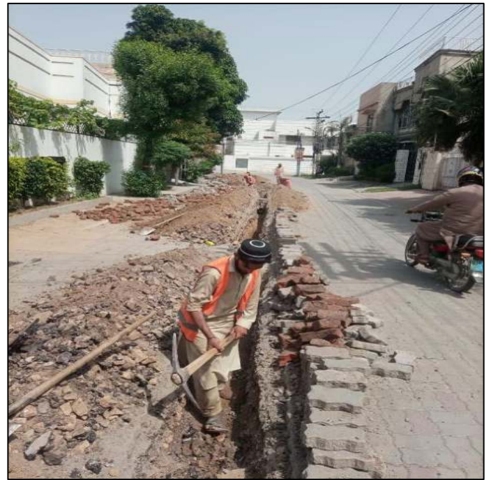
Picture 55: Excavation for laying 90mm HDPE (UC Model Town)
