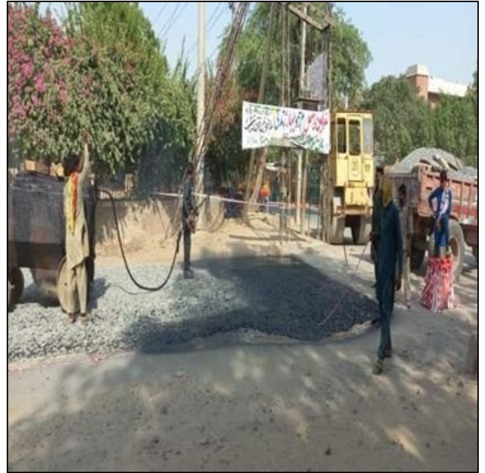
Picture 18: L-2 36" dia TST work in progress
