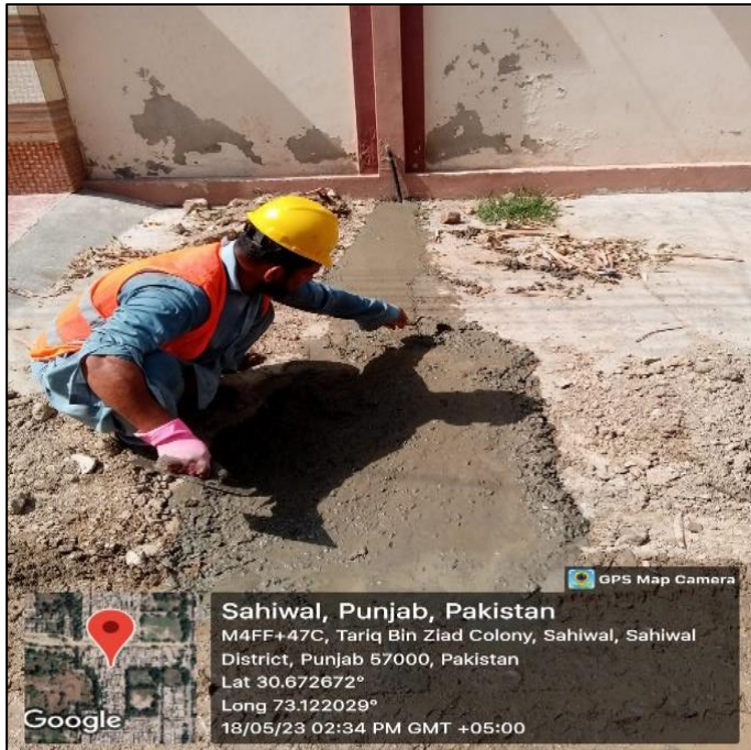
Picture 9: : Restoration of House connection
