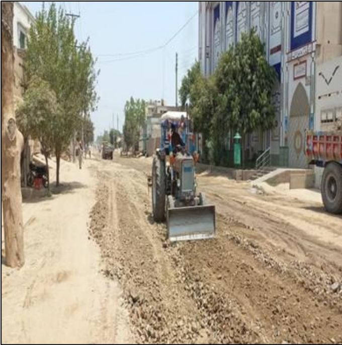
Picture 17: L-2 72" dia sub base spreading in progress
