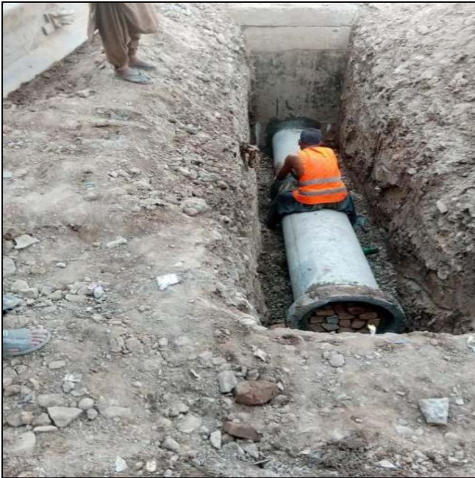
Picture 40: Inlet Pipe Laying in Progress @ Marala Road
