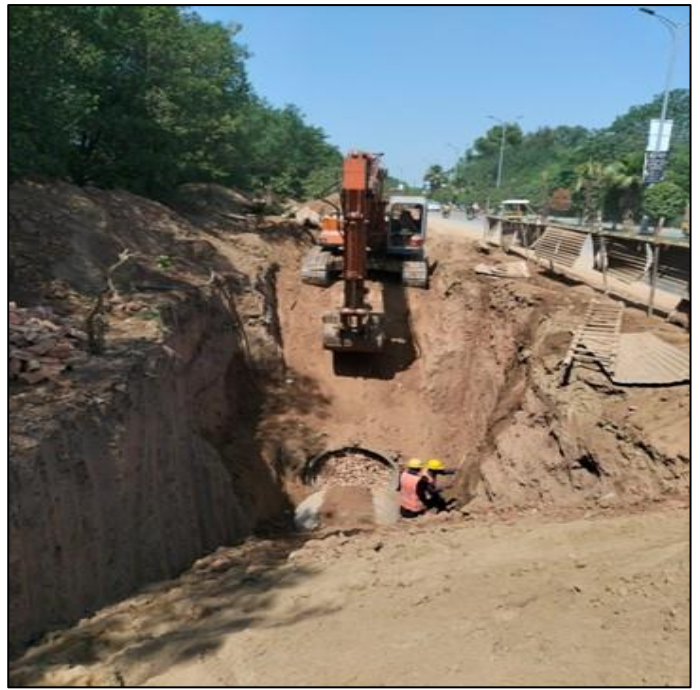
Picture 30: Excavation in Progress for 66" Dia. Sewer Line @ Khawaja Safdar Road
