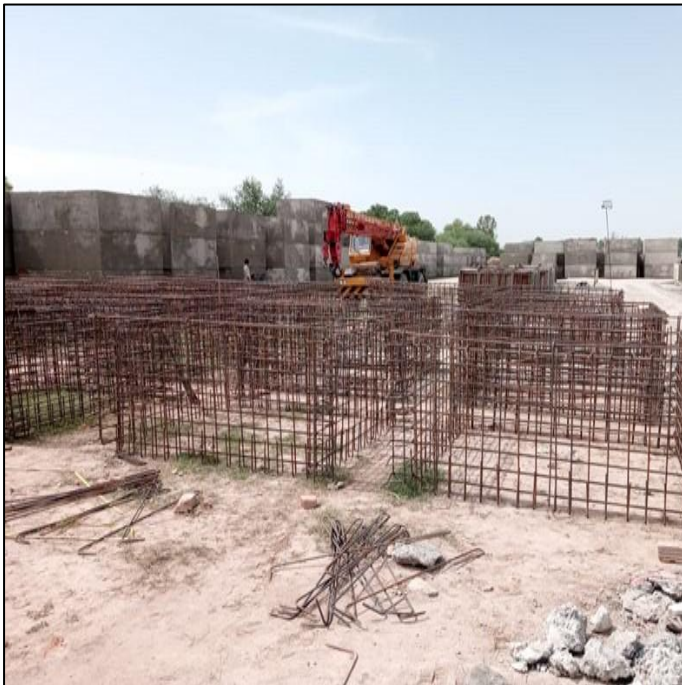
Picture 23: Steel cages for Precast conduit at Camp
