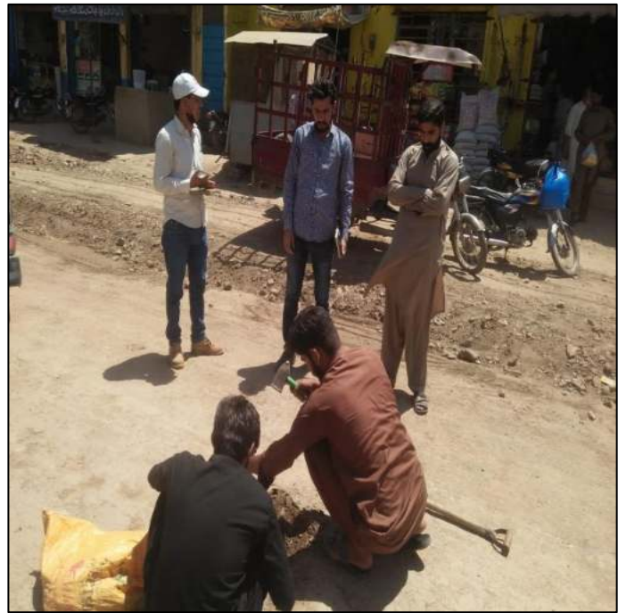
Picture 51: Sample collection for Gradation Test of Sub Base
