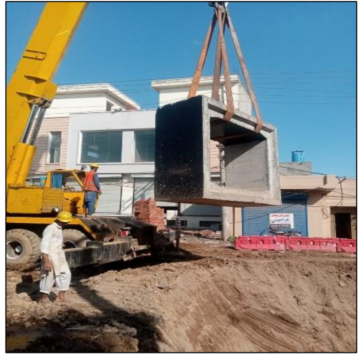
Picture 37: Single Cell Conduit Laying @ Marala Road
