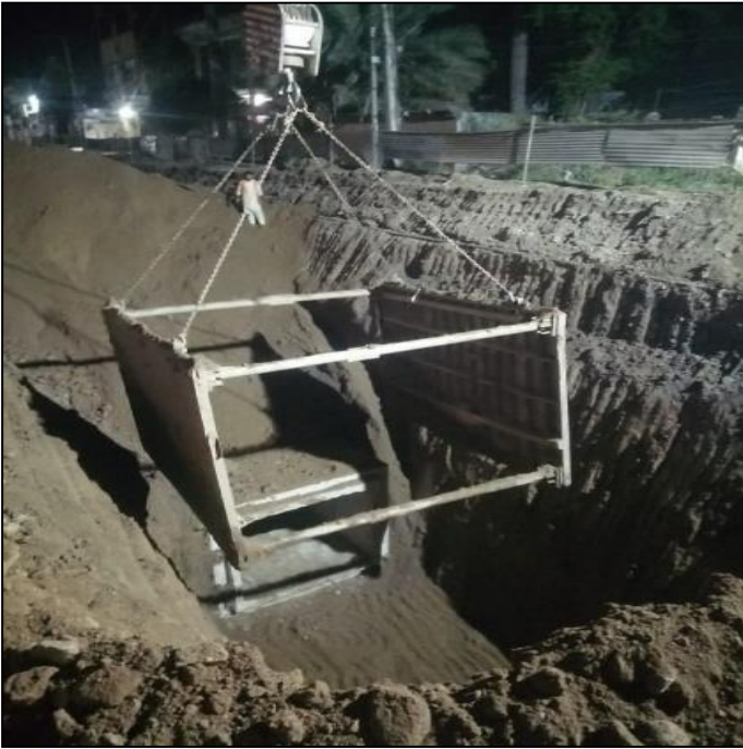
Picture 38: Installation of Safety Box in Progress @ Marala Road
