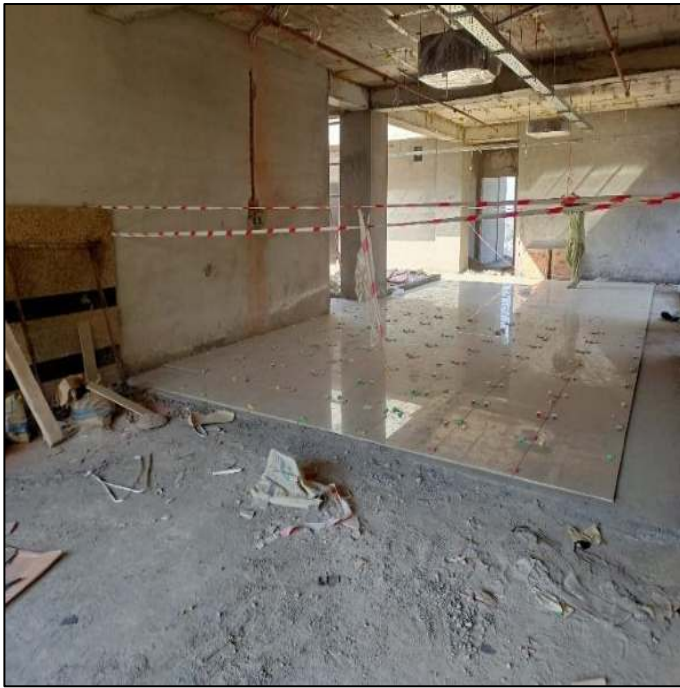
Picture 57: Tile Work 5 th Floor
