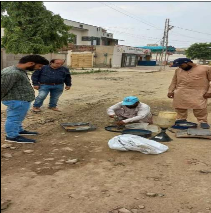
Picture 15: Compaction Test at L-2 27" Dia.
