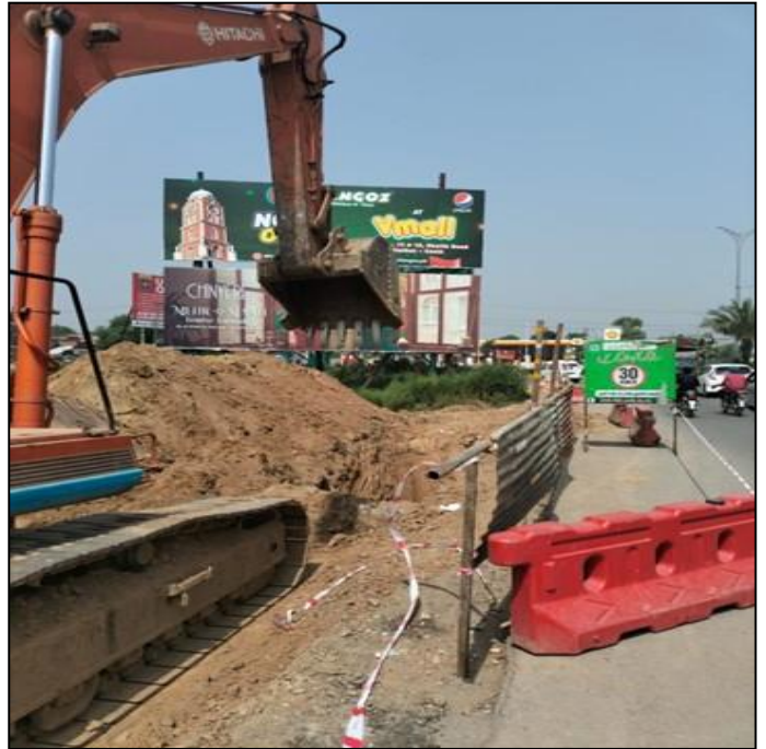
Picture 32: Excavation for Laying 60" Dia. Sewer @ Khawaja Safdar Road
