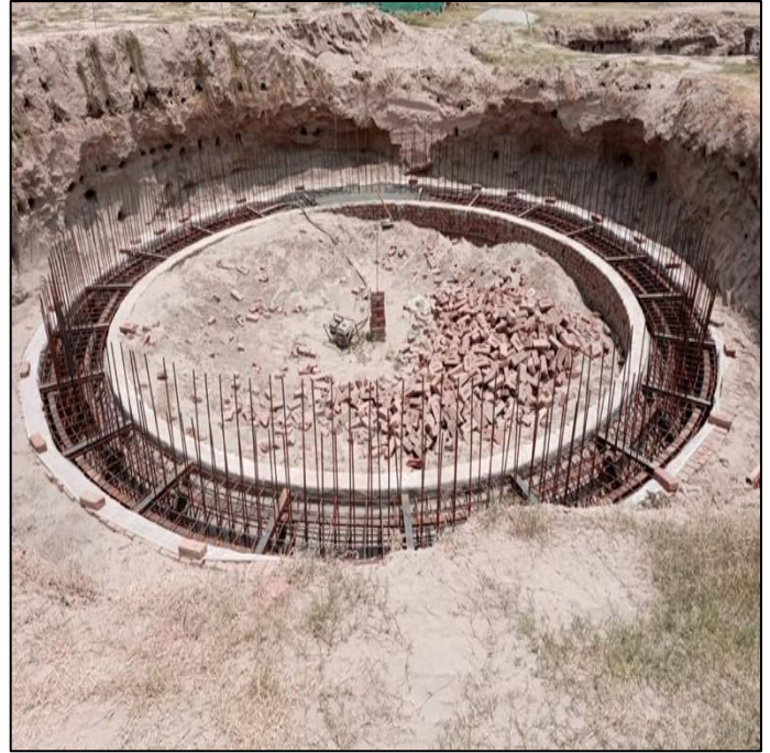
Picture 22: Reinforcement and fixation of cutting edge of wet well curb
