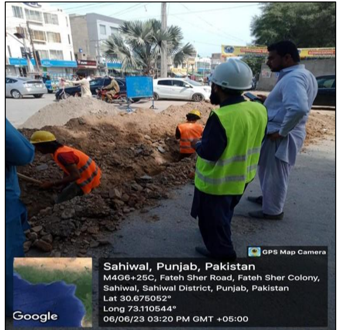
Picture 10: Excavation for HDPE pipe laying at Fateh Sher Road
