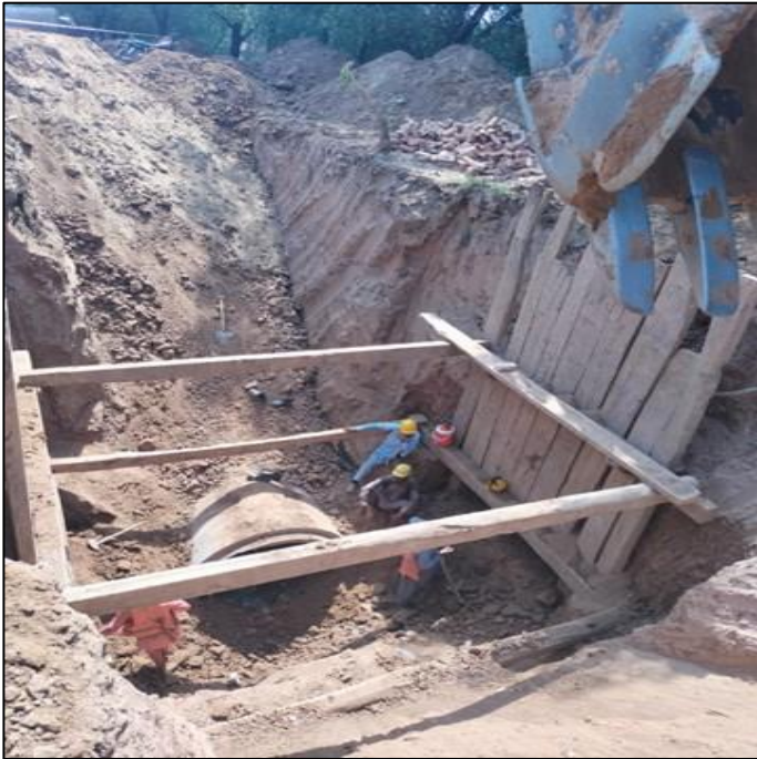
Picture 31: MH 84 Excavation Work in Progress @ Khawaja Safdar Road
