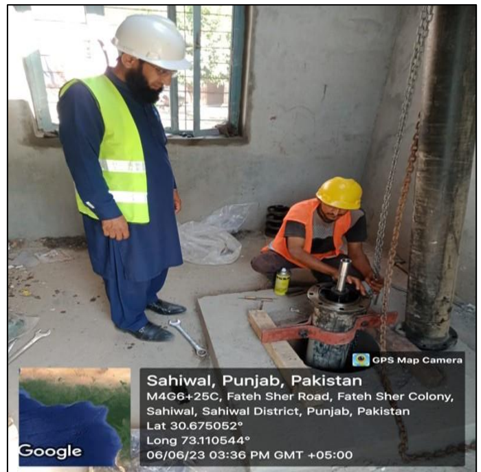
Picture 12: Lowering of Machinery at Fateh Sher Colony P-29
