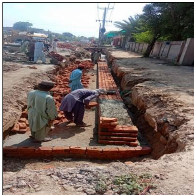
Picture 28: Construction of Drain along the Model Road is in Progress
