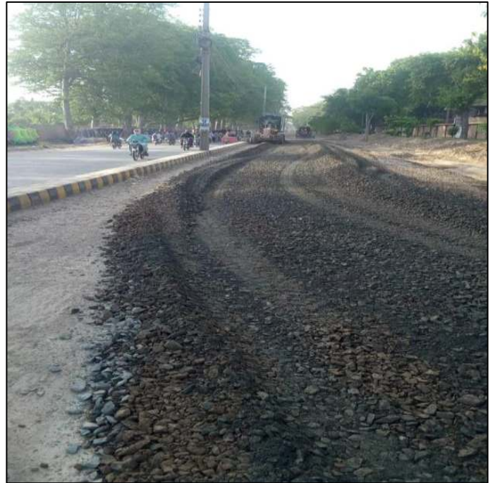
Picture 62: Mixing of Sub base before laying
