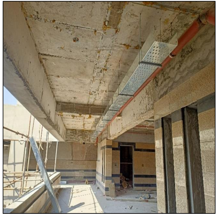
Picture 58: Cable Tray Installation & Cladding Work at 5 th Floor
