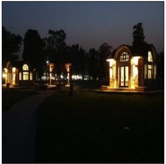
Picture 6: Fixing of Lights in Kiosk 01 & 02 at Gulshan Iqbal Park
