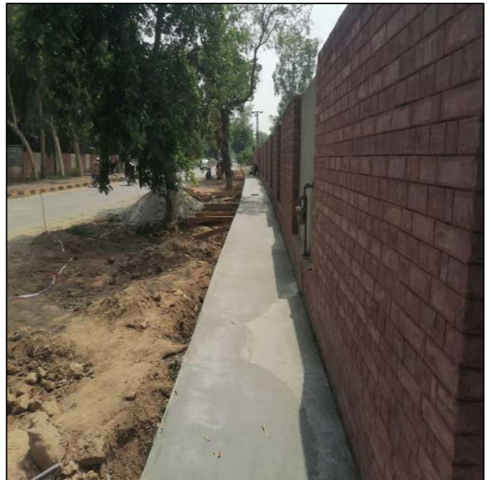
Picture 64: Iqbal Road drain top slab Pouring concrete in progress
