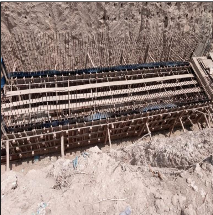
Picture 19: Formwork fixing at 7 x 6.5ft conduit in progress
