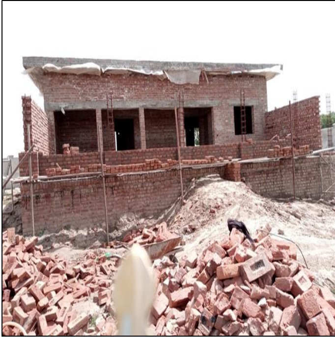
Picture 21: Brickwork in superstructure of office building in progress
