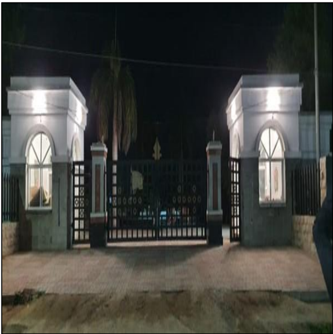
Picture 7: Lights of Security & Ticketing Rooms of Gulshan Iqbal Park
