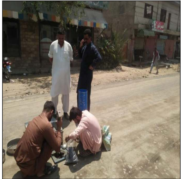
Picture 45: WBM FDT in Progress @ Marala Road
