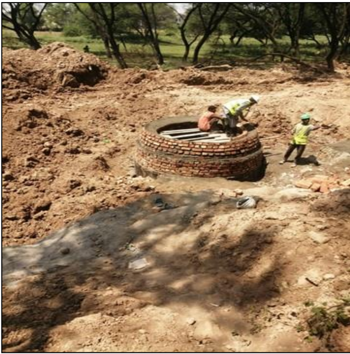
Picture 29: Brick Masonry Work in Progress @ Khawaja Safdar Road
